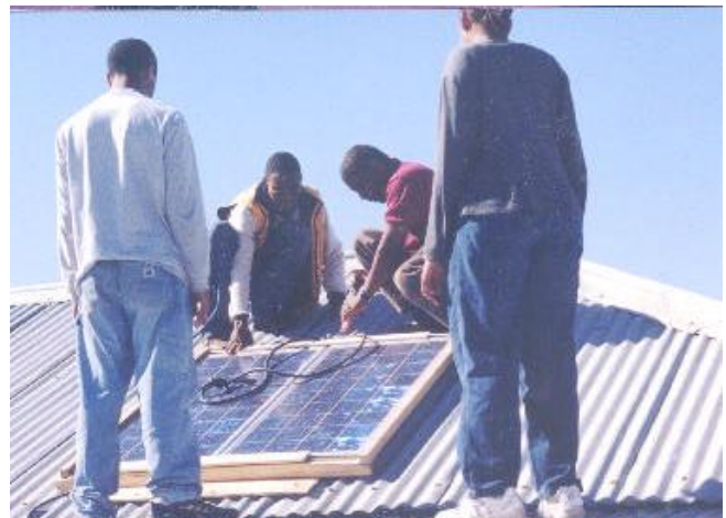
FIGURE. 2 INSTALLING SOLAR PANELS ON THE ROOF OF HOME [3]
