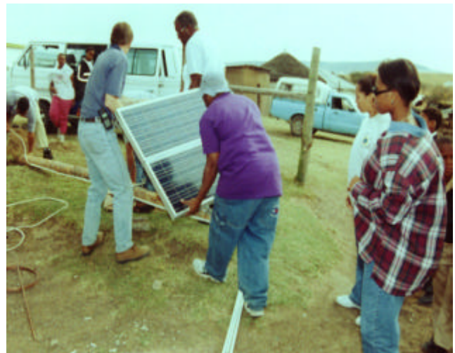
FIGURE. 1 REEP STUDENTS INSTALLING 100-WATT DC SYSTEM IN SOUTH AFRICAN RURAL VILLAGE [3]
