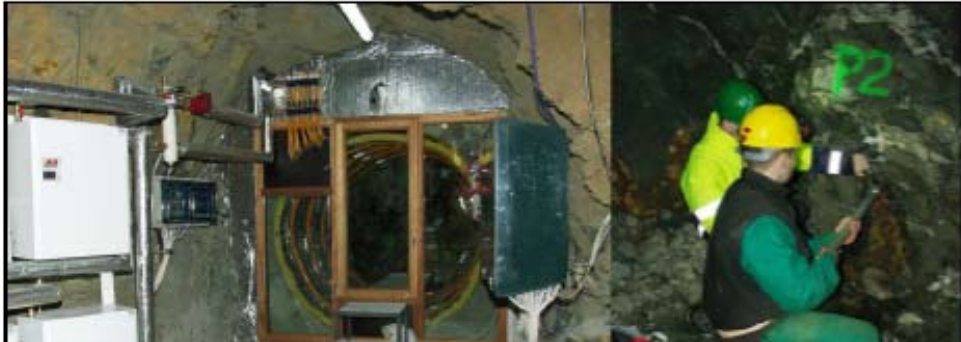
Figure 8: TIMODAZ experiment (left) and bentonite plugs sampling (right)
